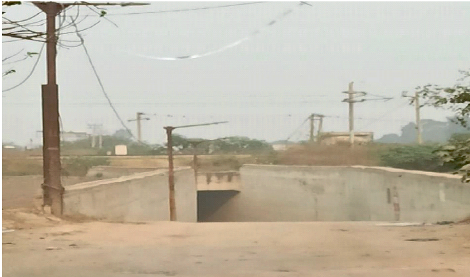
Image 2: Nasrali underpass, the only alternative to the level crossing.
